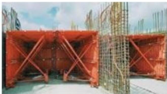
**Tunnel Formwork System**
